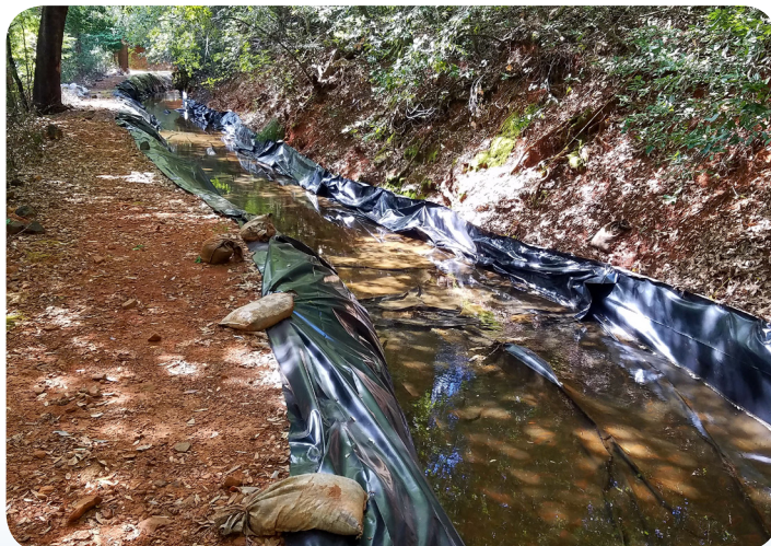
Plastic sheeting is used to reduce water seepage on parts of the Forbestown Ditch.
