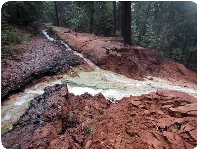
A blowout, breached section of the Forbestown Ditch, January 2017.
